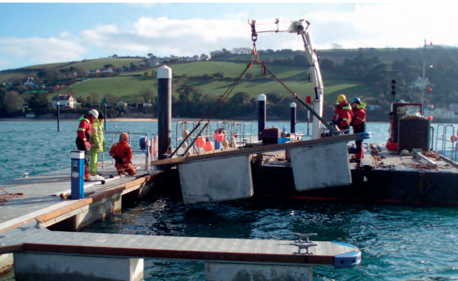
Moorings Team fitting the new finger berths onto Normandy Pontoon
